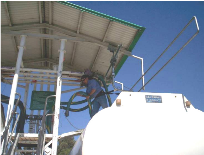
The operator lifts the hoses over to the tank
